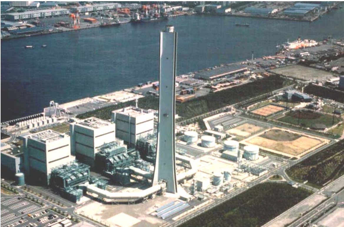
Photo 1. Bird's eye view of the smokestack of Nanko Thermal Power Plant of KEPCO (By courtesy of KEPCO)
